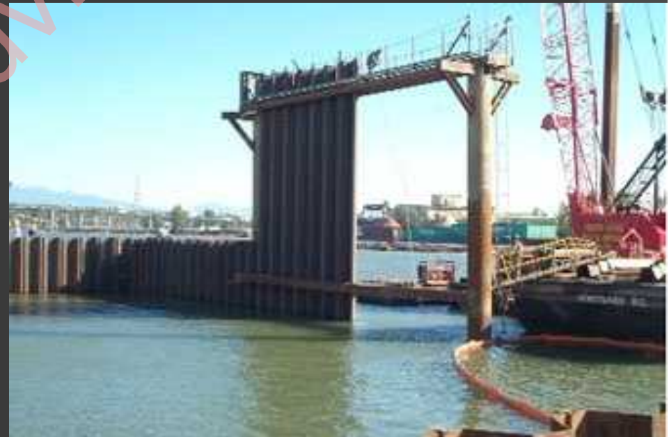
Single sheet pile cofferdam
